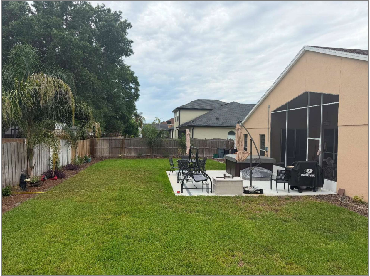
Photo 3 - Exhibit C – Existing Rear Yard Depth
