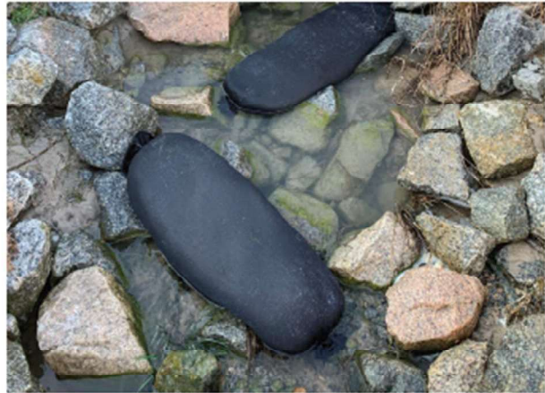
Small ditch installation showing EutroSORB F Filters.
