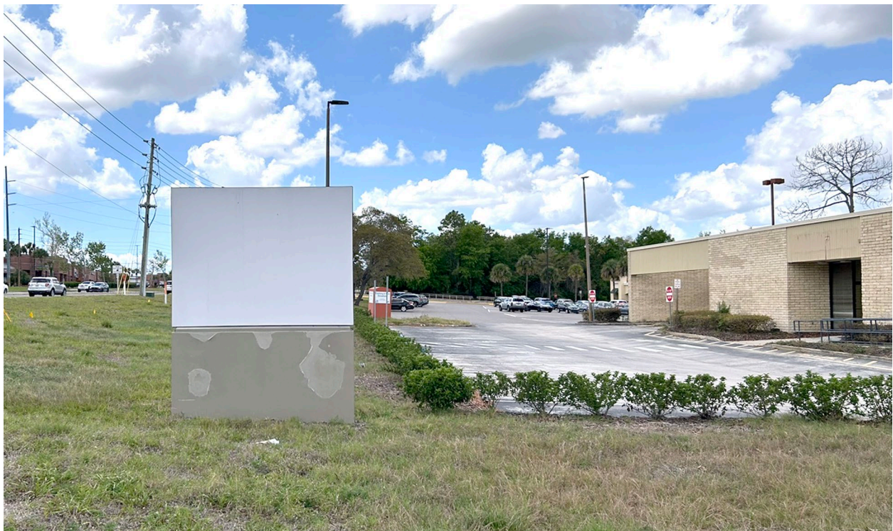
Figure 2 – Existing sign structure previously used by Wells Fargo
