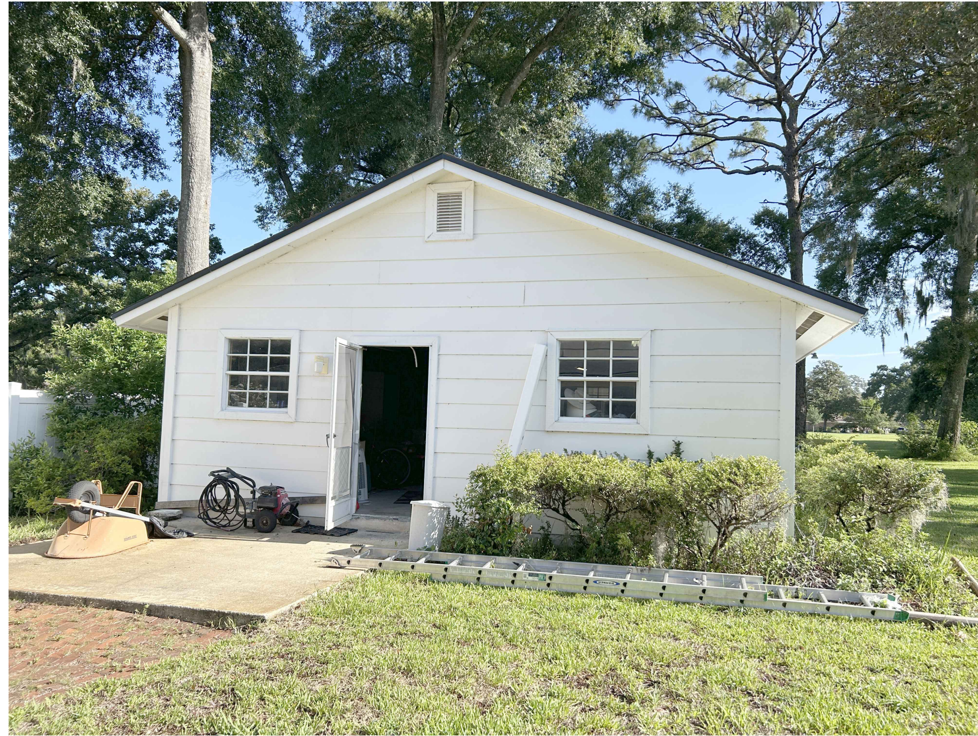
SOUTH ELEVATION PHOTO
