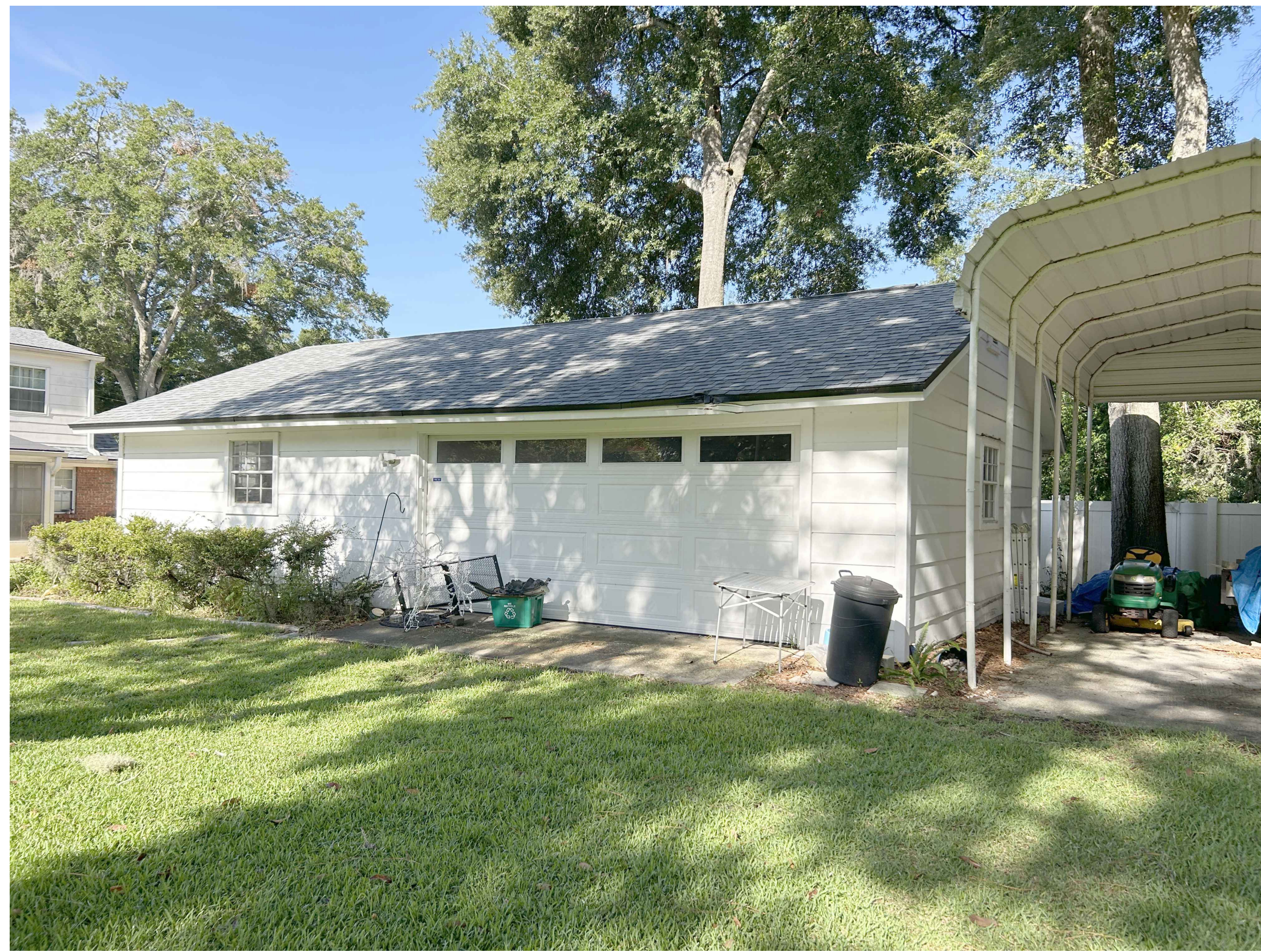
EAST ELEVATION PHOTO
